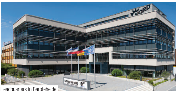
Headquarters in Bargteheide
